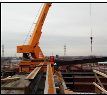
IC-200-2C from previous bridge jobs, took full advantage of the additional reach provided by the IC-200-3D. The Broderson IC-200-3D would be utilized in all aspects of the construction process, from moving the portable matt to the transporting and placement of the I-beams to be used in the construction of the actual bridge decking.
